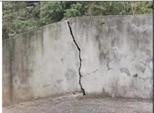
溢洪道边墙破损
