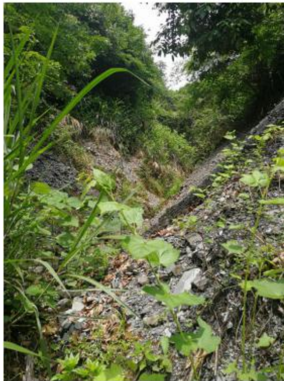
8#刘家组下簸箕废渣堆积现状
